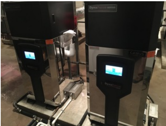
Heating water boiler
