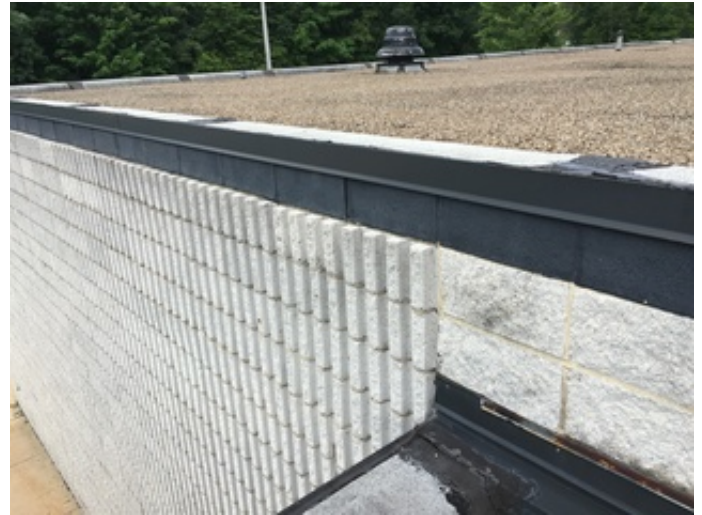
Edge trim and counterflashing
