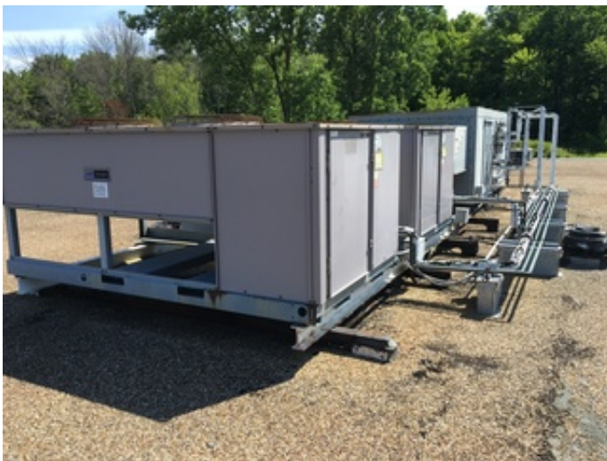
Air cooled condensing unit
