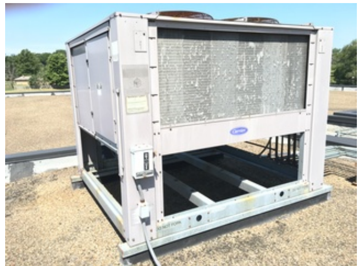
Air cooled condensing unit
