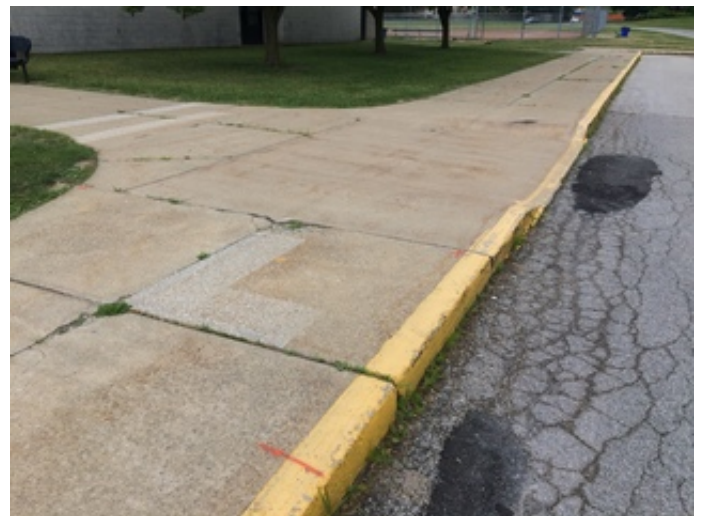
Damaged pavement/walk & non-compliant ramp
