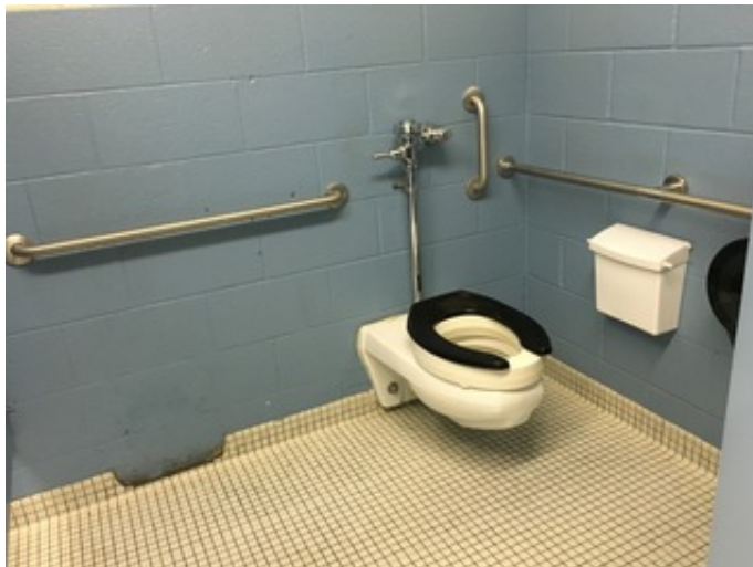
Obstructed grab bar installation
